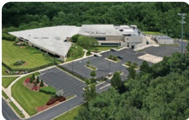
BYTEGRID's Maryland Data Center
